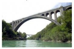
The Solkan Bridge is a famous detached bridge over the Soca River in Solkan on the Bohinj Railway Jesenice - Nova Gorica. The bridge has the longest stone arch in the world and the longest stone arch between railway bridges. The main arch used 4,533 precision machined rock shell stones from the quarry near Nabrežina.
